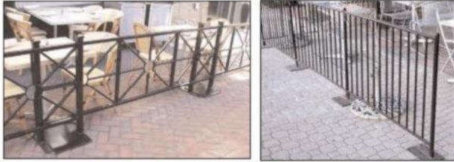
Examples of open-style sectional fencing that acts as a pedestrian barrier to enclose outdoor dining areas.
